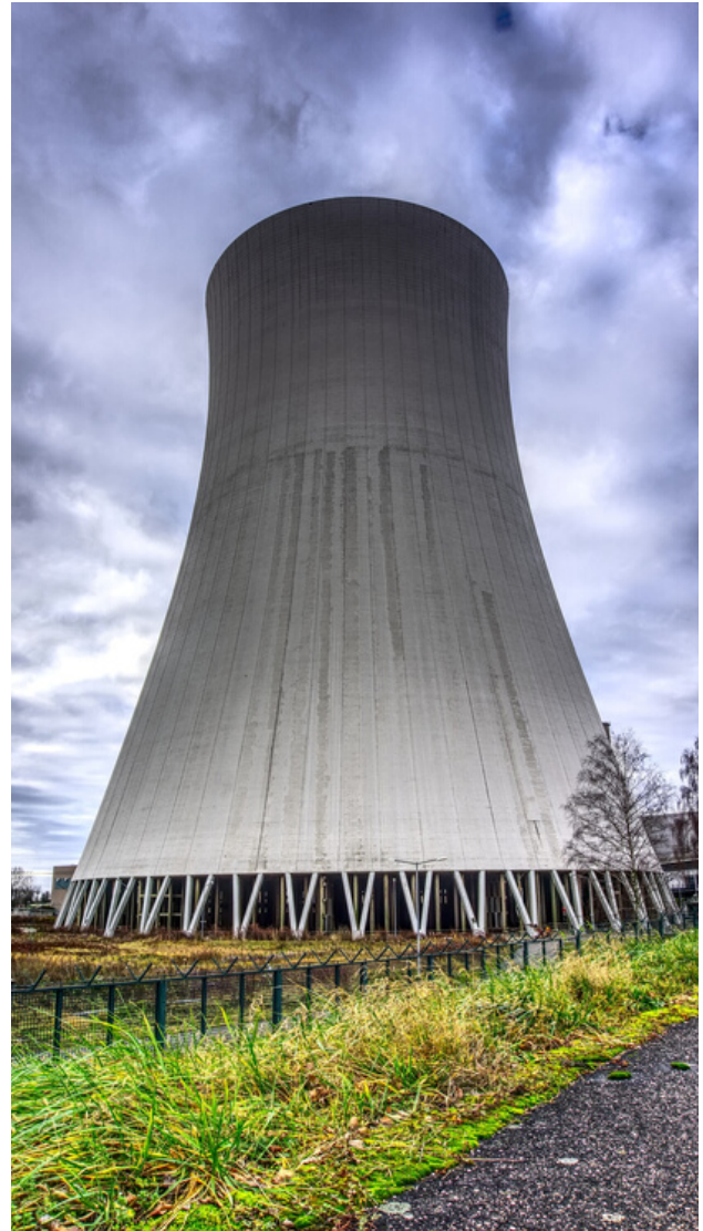
COOLING TOWER NUCLEAR POWER PLANT
